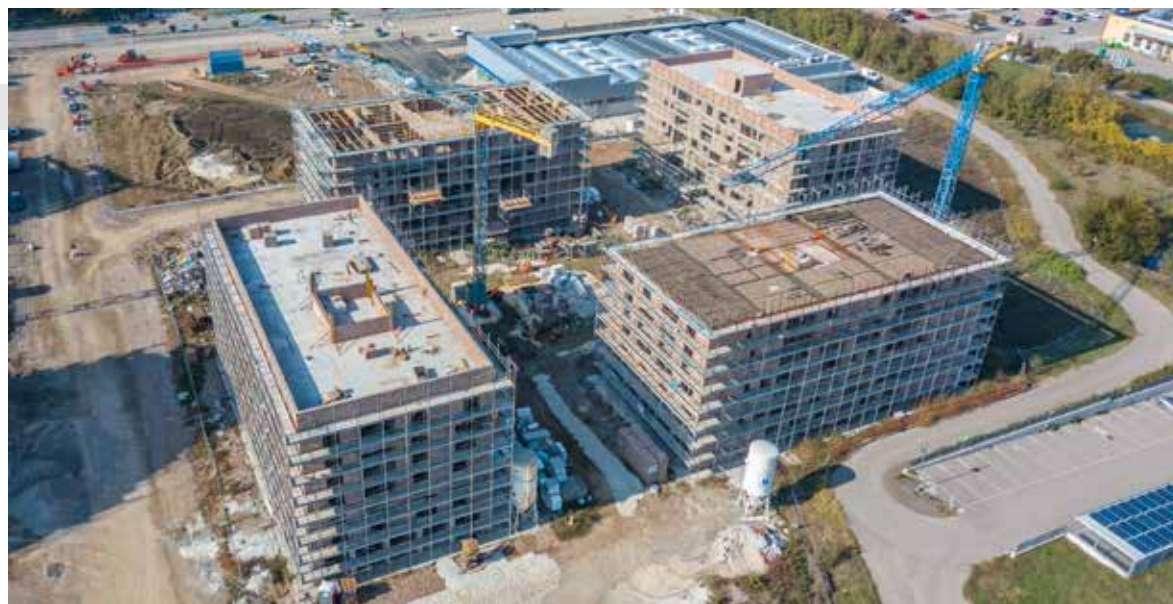
Social Housing 80 alloggi a Granarolo (BO) - 2020
