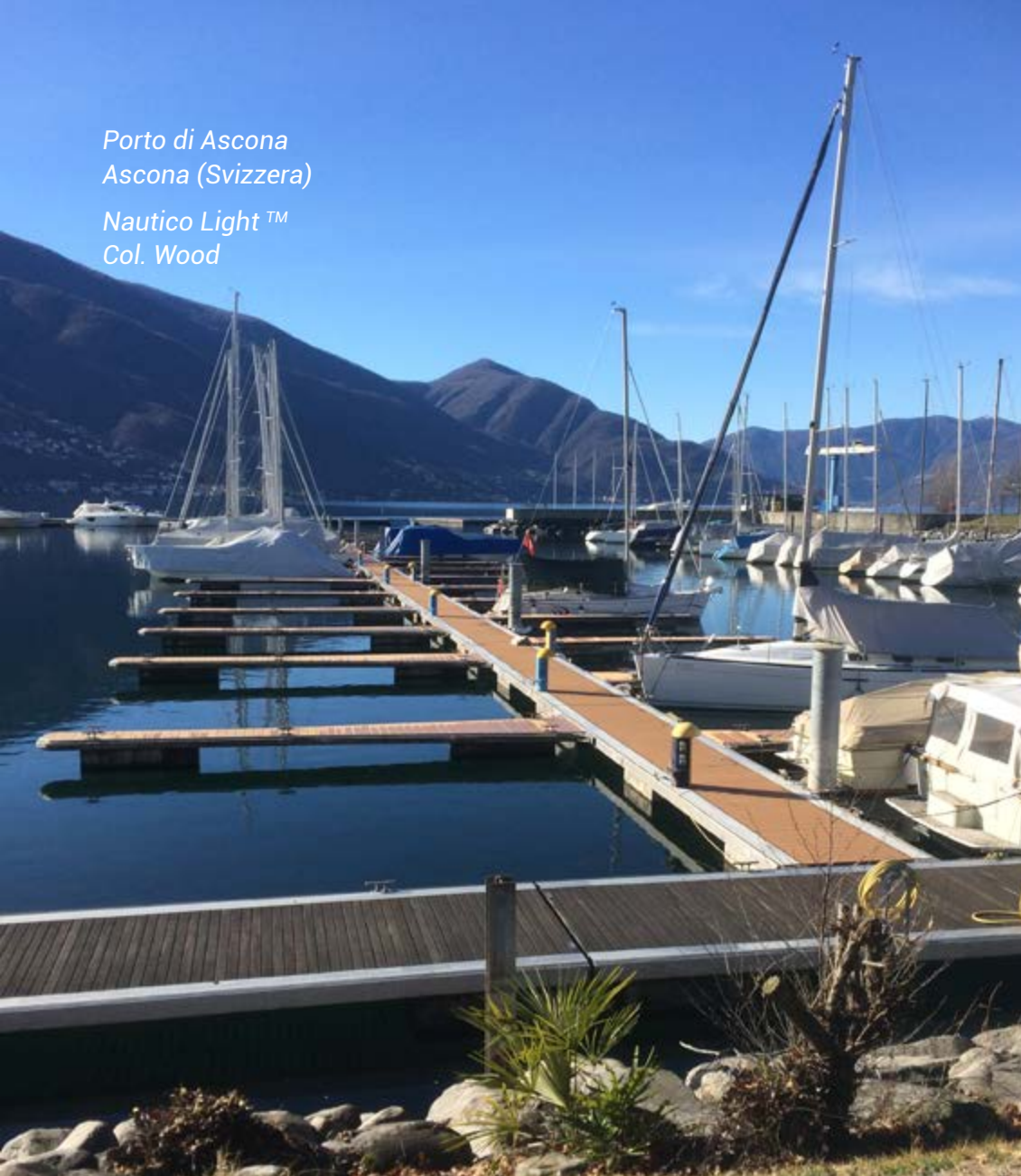
Ponti e pontili Bridges and pontoons
